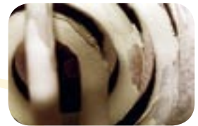
Heating coil before
